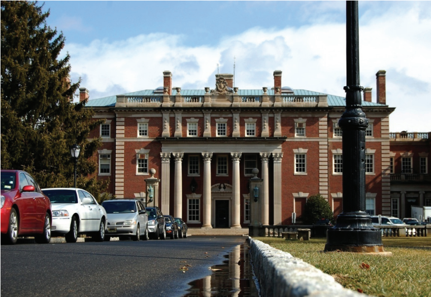
Figure 2: The Mansion as university building, main façade. The building now serves as offices and classrooms on the Florham campus of Fairleigh Dickinson University. Photo courtesy of Dan Landau Photography
