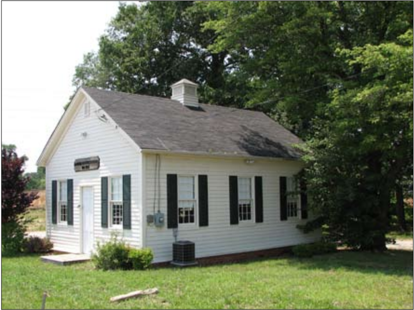
Figure 3: Laurel Grove School, Fairfax County, Virginia, 2007. Photo by Linda Sargent Wood.
